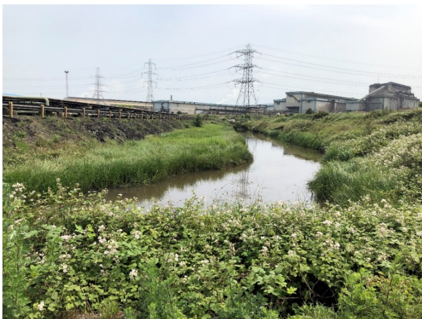
Figure 2: Lackenby Channel looking south.
